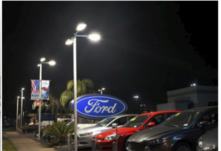
Long Beach Port — LED Shoebox light replacement
